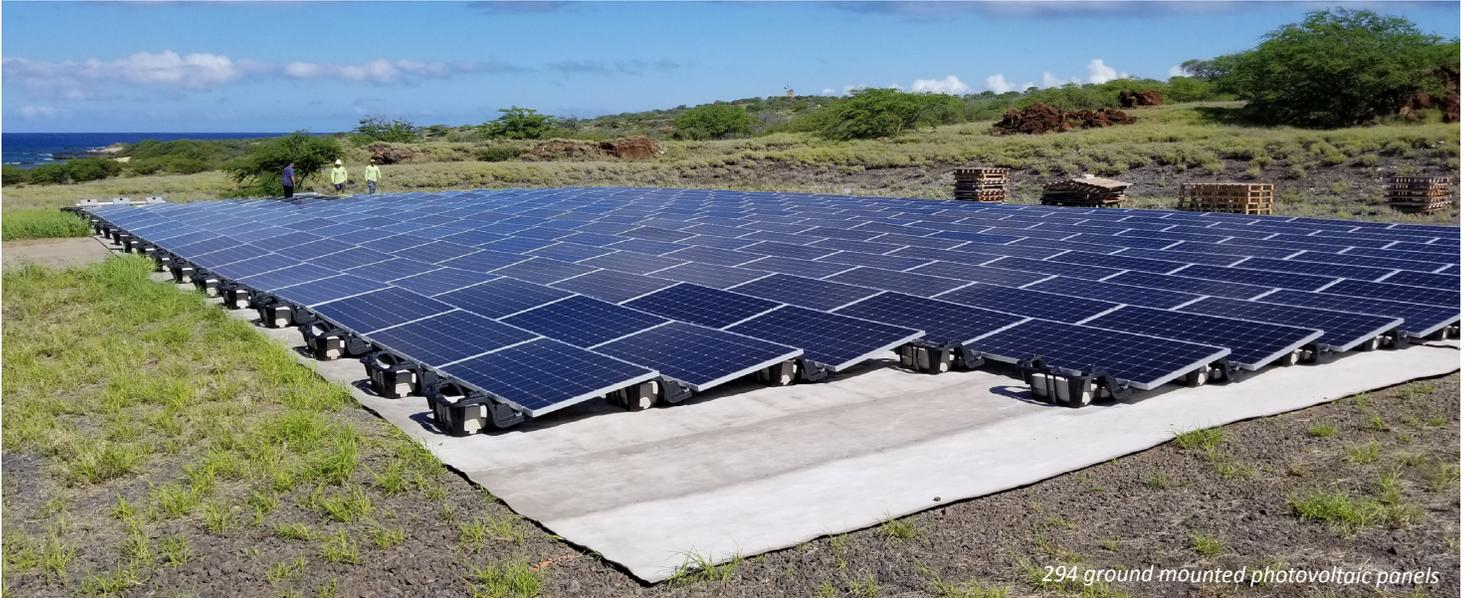
294 ground mounted photovoltaic panels
