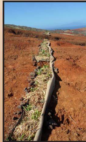
Wattles (left) and Raised Planting Bed Corridors (right).
