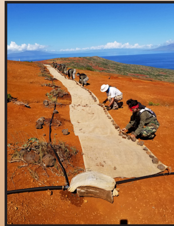
Wattles (left) and Raised Planting Bed Corridors (right).
