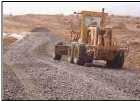
Construction of Kuamo'o Road
