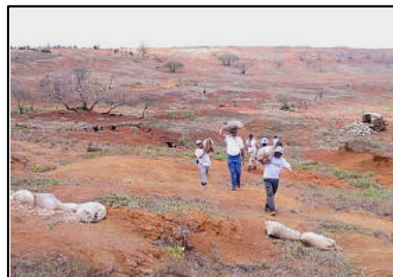
Erosion Control Work at Luamakika
