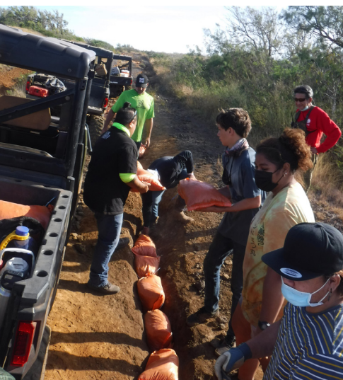
▲ Hui o Na'ulu student volunteers placing gravel bags along eroded sections of the K-1 road
