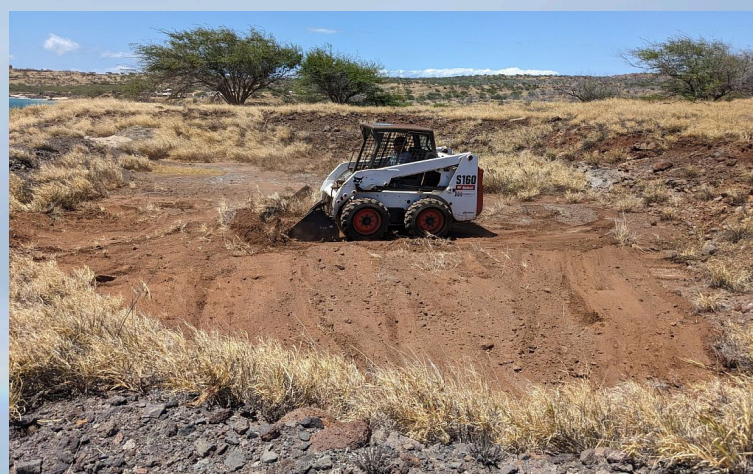
▲ The silt retention pond being excavated
