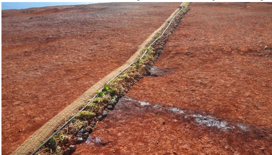
The finished wattle product with native plants on irrigation in the project site
