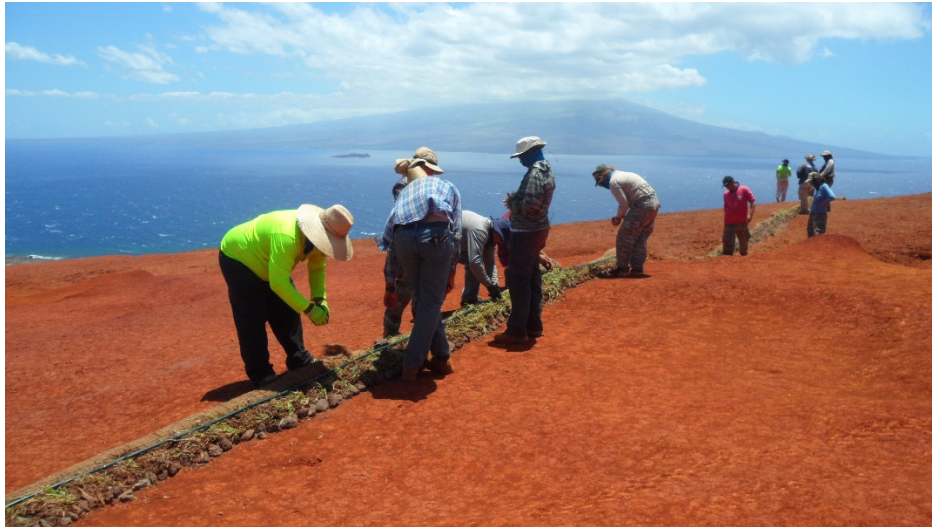
Kamehameha School Teachers installing a wattle with native plants and irrigation.
