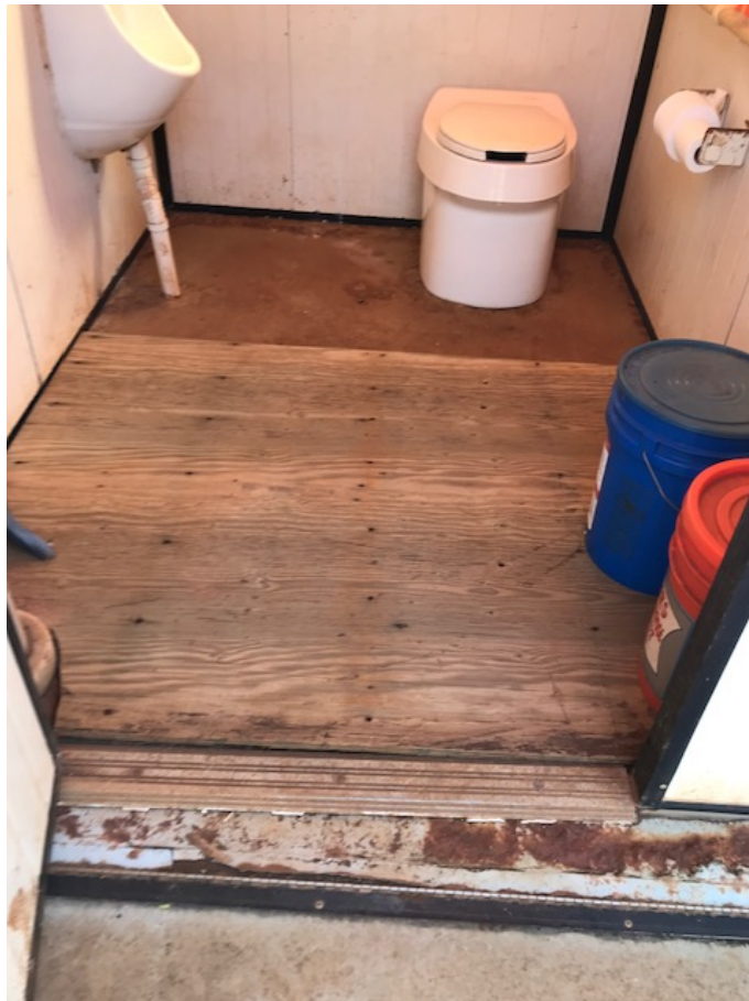
Reinforced floor of lua on Hawai'i Island-side, left
