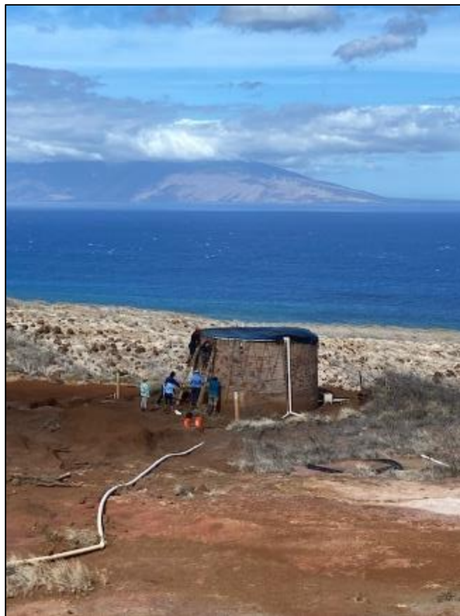
Figure 1. Wailuna - Installed Mesh Cover On Water Tank (photo courtesy of Momi)
