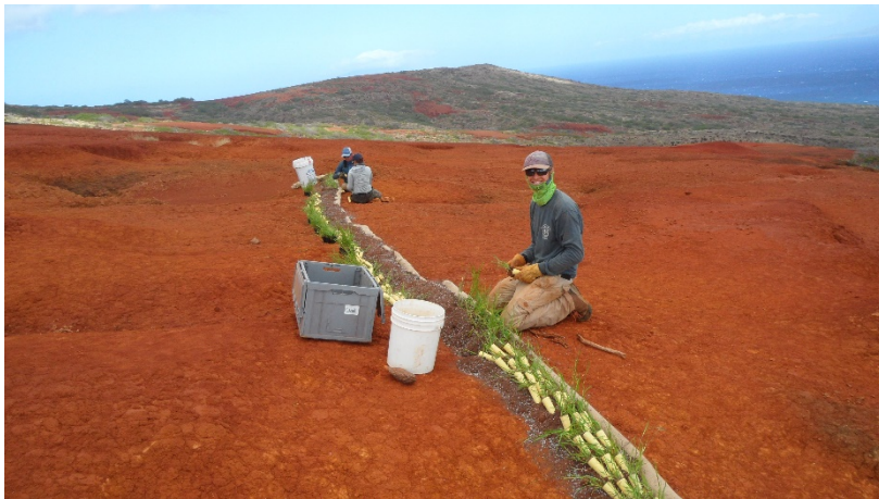
Planting pili grass in the soil mixture in the wattle corridor
